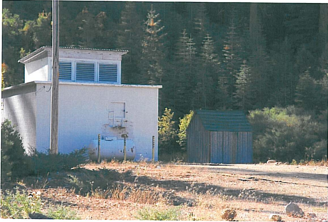
French Meadows - Hell Hole Tunnel Inlet Gatehouse
