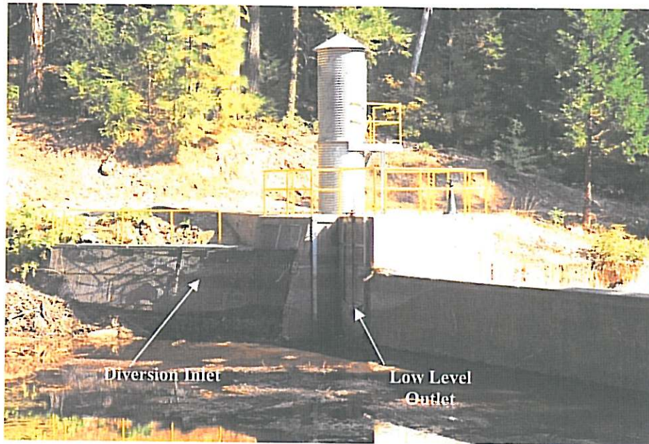
North Fork Long Canyon Diversion - Downstream Side
