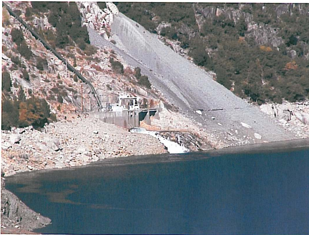
French Meadows Powerhouse
