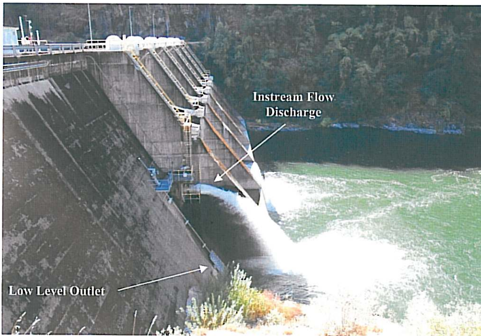
Ralston Afterbay Dam - Downstream
