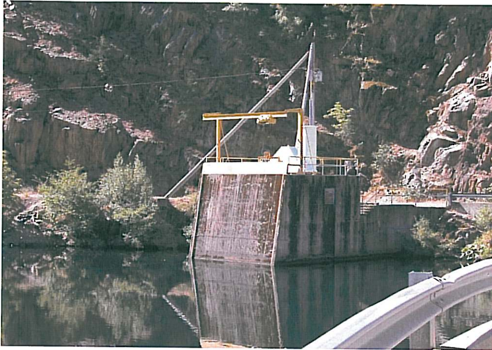
Middle Fork - Ralston Tunnel Inlet Structure
