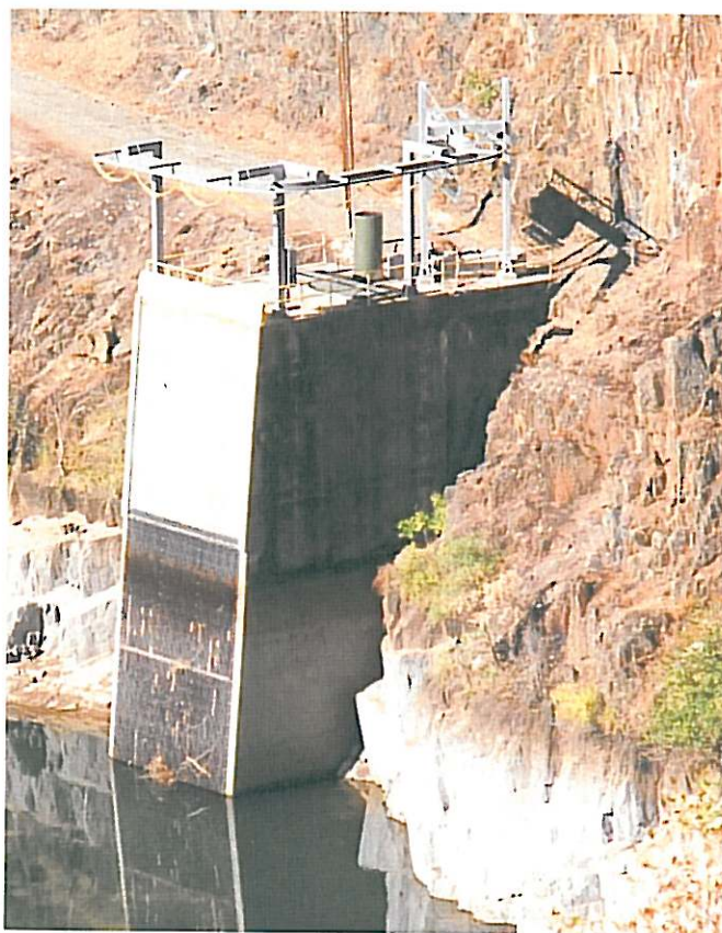
Ralston-Oxbow Tunnel Inlet Structure
