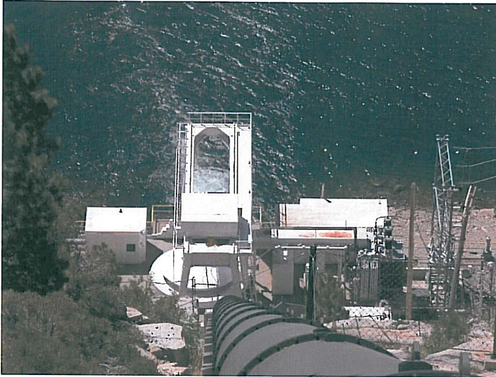
French Meadows Powerhouse
