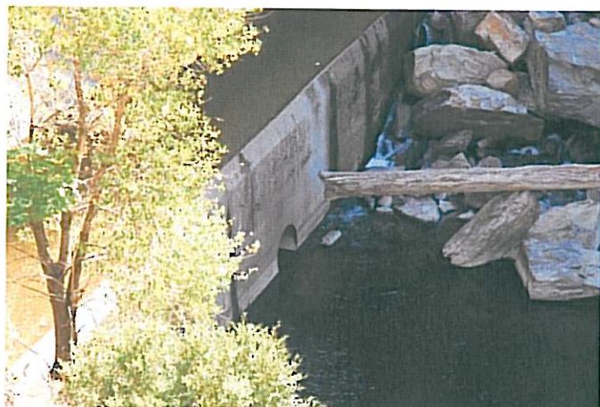
Interbay Dam Low Level Discharge
